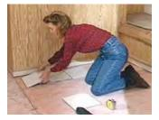
Tile looks best if it's laid out in straight line and square to the walls. That requires a bit of layout prior to installation.
